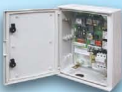
Electrical power panel with Elpro 10 exp
